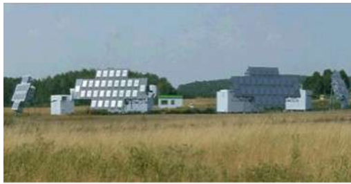
Figure 6.2.9 - transmitting - receiving antennas
